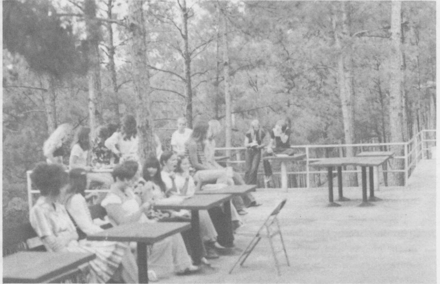
Terrace built out over an incline (an extension of the dining hall)
