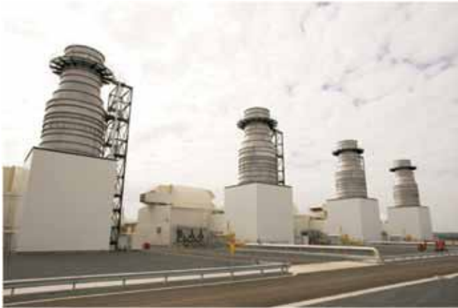
Uranquinty Power Station, Australia
