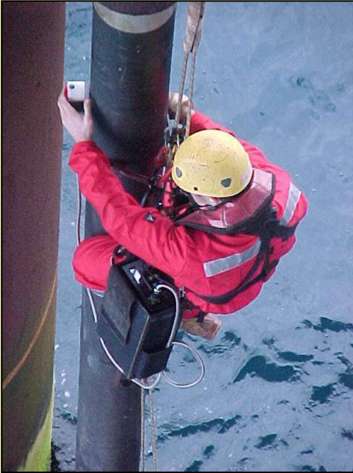
Inspect through coating, rope access
