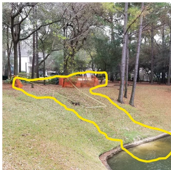
Silt has traveled from the sink-hole above under-ground to the lake visible in the photograph. The area below the sink-hole also is also in danger of collapsing.
