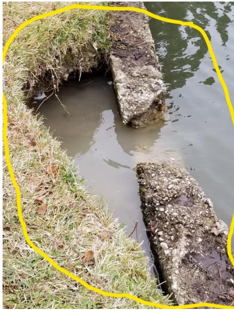
The concrete bank-head has broken and is starting to erode. It has gradually become as larger as no work has been done to fix the problem.
