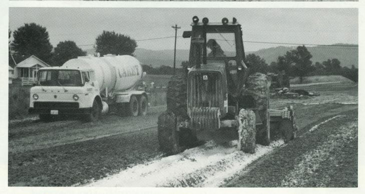
The combination of a Howard Rotavator with todays modern tractor with multi speed or hydrostatic transmission makes a low cost mixer package.
