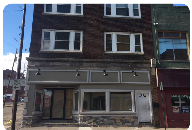
We helped fund the facade renovations of 40 N. Wyoming St., located at the corner of Green and Wyoming Streets.
