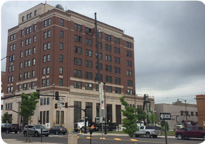
DHD Realty continued renovations on 101 W. Broad St. (the former HNB Bank Building). Nearly $6.5M of private funding was invested in capital improvements within the Main Street District in 2017.
