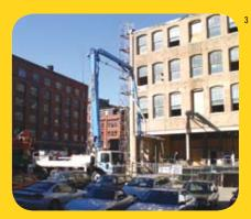
Lighter and more resilient. Putzmeister's "smart design" boom incorporates welding seams below the edge of maximum stress. The boom is engineered to offer the flexibility to adapt to different loads and features more straight pipe for a less stressful concrete flow and longer wear on parts. The Multi-Z configuration handles space restrictive areas and can pump even if the boom is not fully extended.
