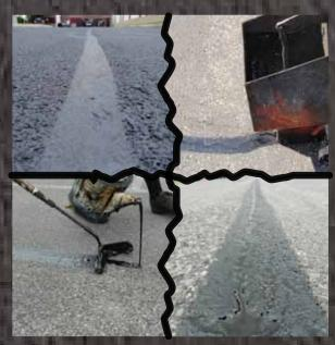
Hot Pour Crack and Joint Sealants for Asphalt Pavements and Portland Cement.
