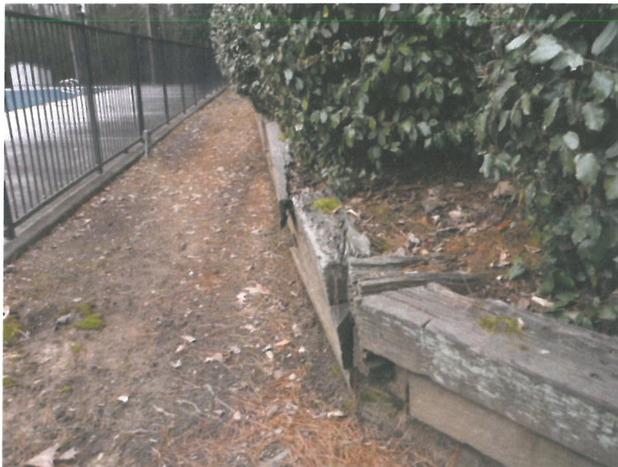
Aging retaining wall
