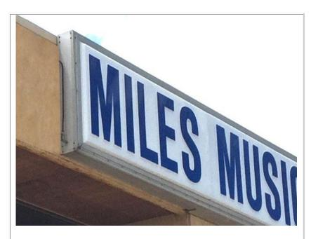
Firstly, the thermo form face was removed, then the TS22 frame was screwed to the front of the light box.
