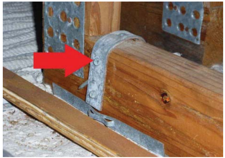
#4 ROOF TO WALL ATTACHMENT OPPOSITE SIDE
