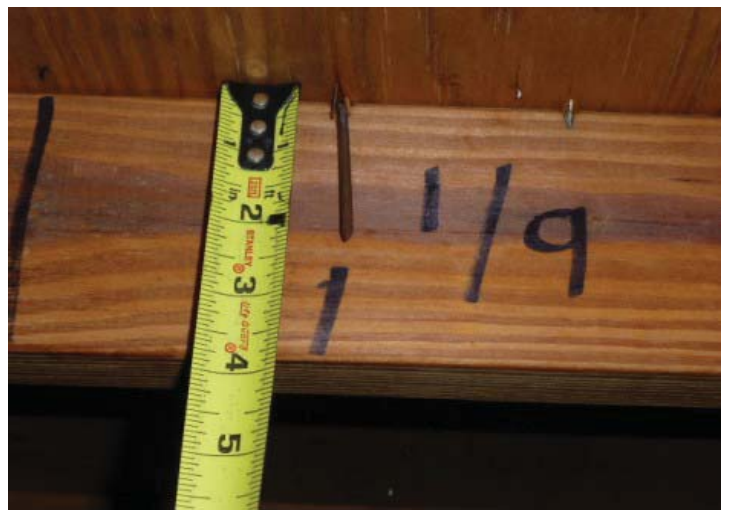
#3 ROOF DECK ATTACHMENT 8d NAILS
