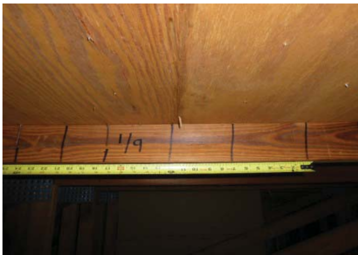
#3 ROOF DECK ATTACHMENT 6" X 6" NAIL SPACING
