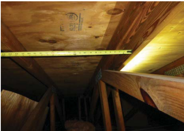
TRUSS/RAFTER SPACING
