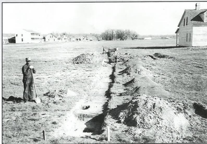
1950 excavation behind Quarter's A in search of Fort John's foundation.
