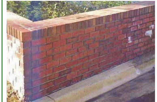
Before & After Efflorescence Removal
