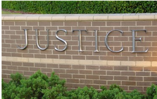
Before & After Brick Restoration
