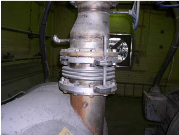
Figure 10. LS 12 Blower, Compressed Bellows at Intake Nozzle.
