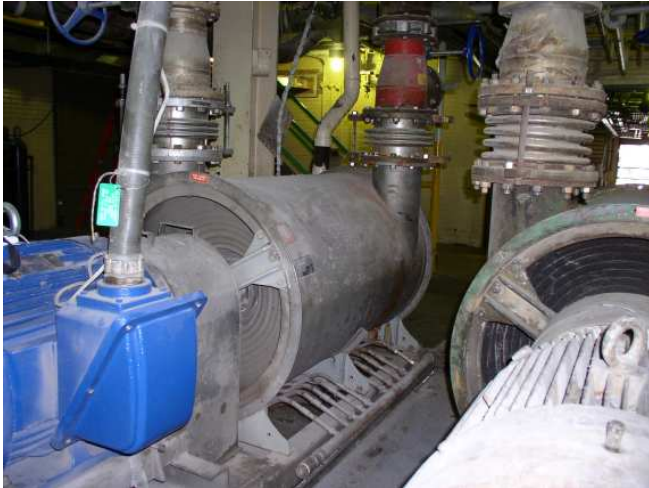
Figure 1. Photo of Multi-Stage Centrifugal Blowers.
