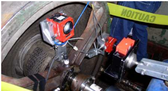
Figure 37. Permalign Ref 7 Setup on Blower and Motor.
