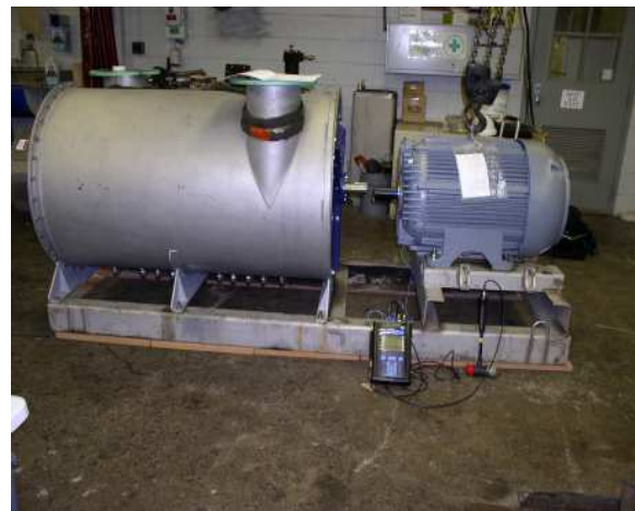
Figure 18: Blower & Skid Supported on Cork in the Maintenance Shop During Modal Test.
