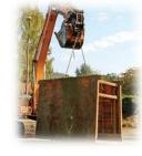
from **cave-ins**. Contractors must **safeguard workers** and commit to **protecting** them from **cave-ins** by properly **shoring** and **sloping** trench walls or by using **shields** (*trench boxes*) to guard from **trench walls** that could **collapse** unexpectedly.
