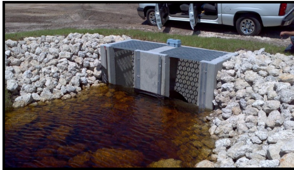
Cypress Creek Flow-way Restoration
