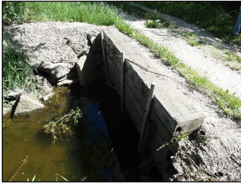
Culverts under Maintenance access drive east of C.-P.R.R tracks, spring, 2013
