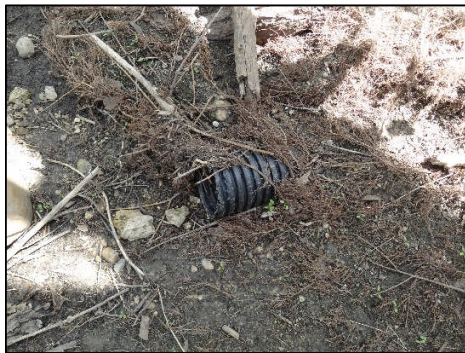
Drain tile outlets into Somers Branch from the south field at Gitzlaff, above and right
