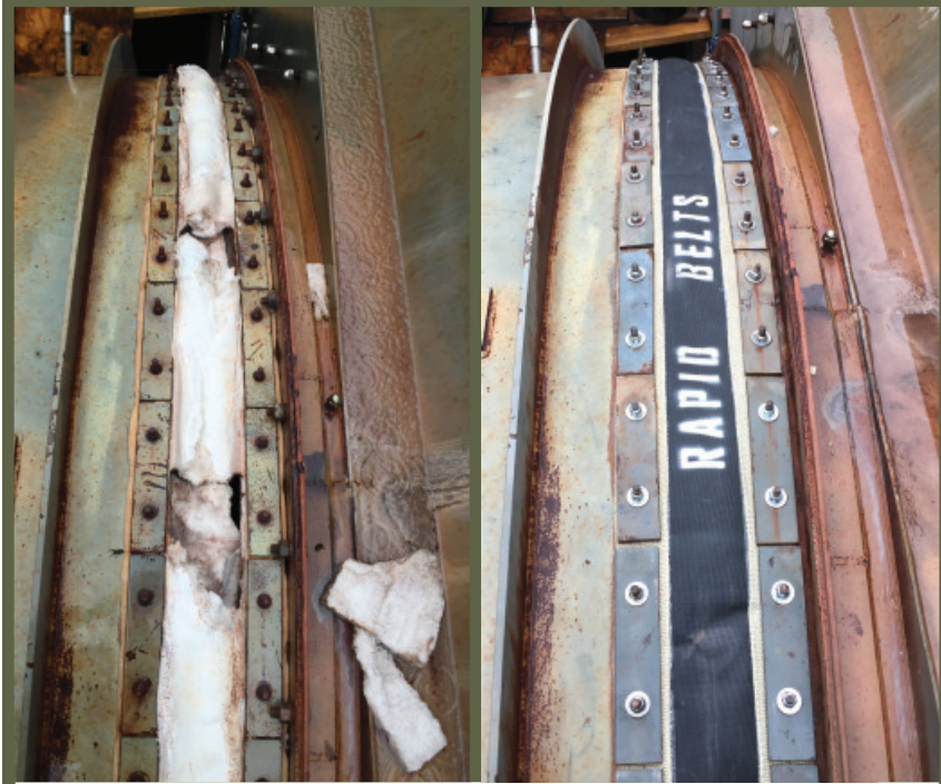
Complete Expansion Joint Upgrades
