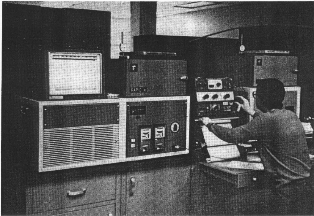
FIGURE 2 - THE RAPID-K THERMAL CONDUCTIVITY INSTRUMENT.
