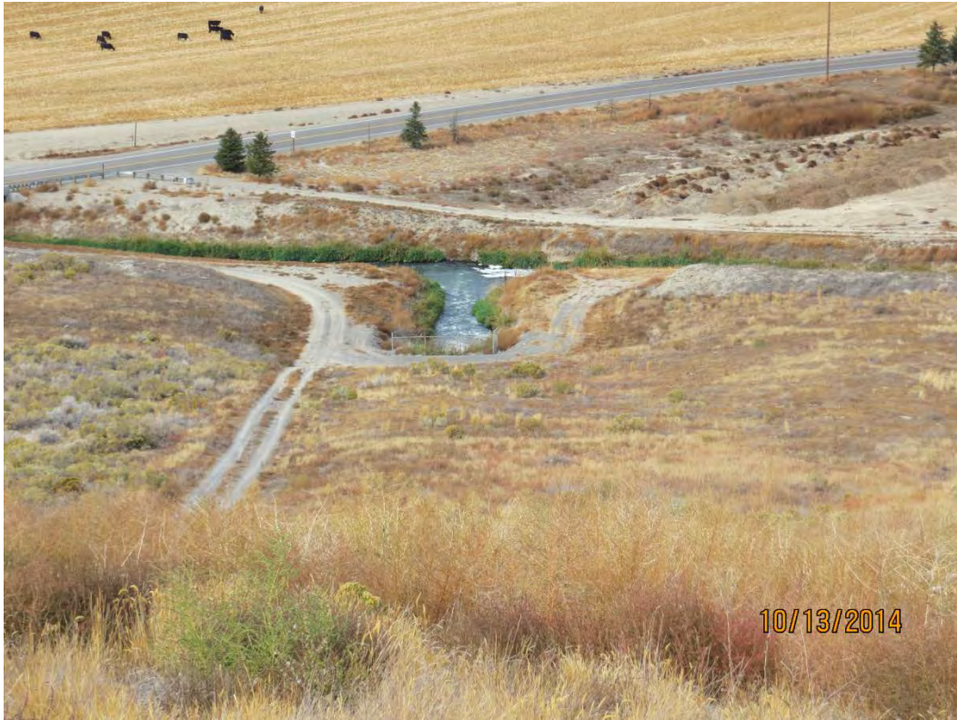
PHOTO 3 BURIED CHUTE AND STILLING POOL LOOKING DOWNSTREAM
