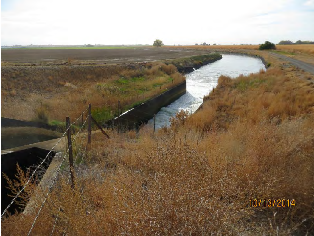
PHOTO 1 CHECK DROP AND STILLING POOL
