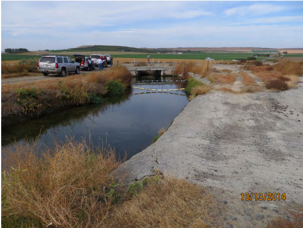
PHOTO 1 WASTEWAY CHUTE INLET STRUCTURE
