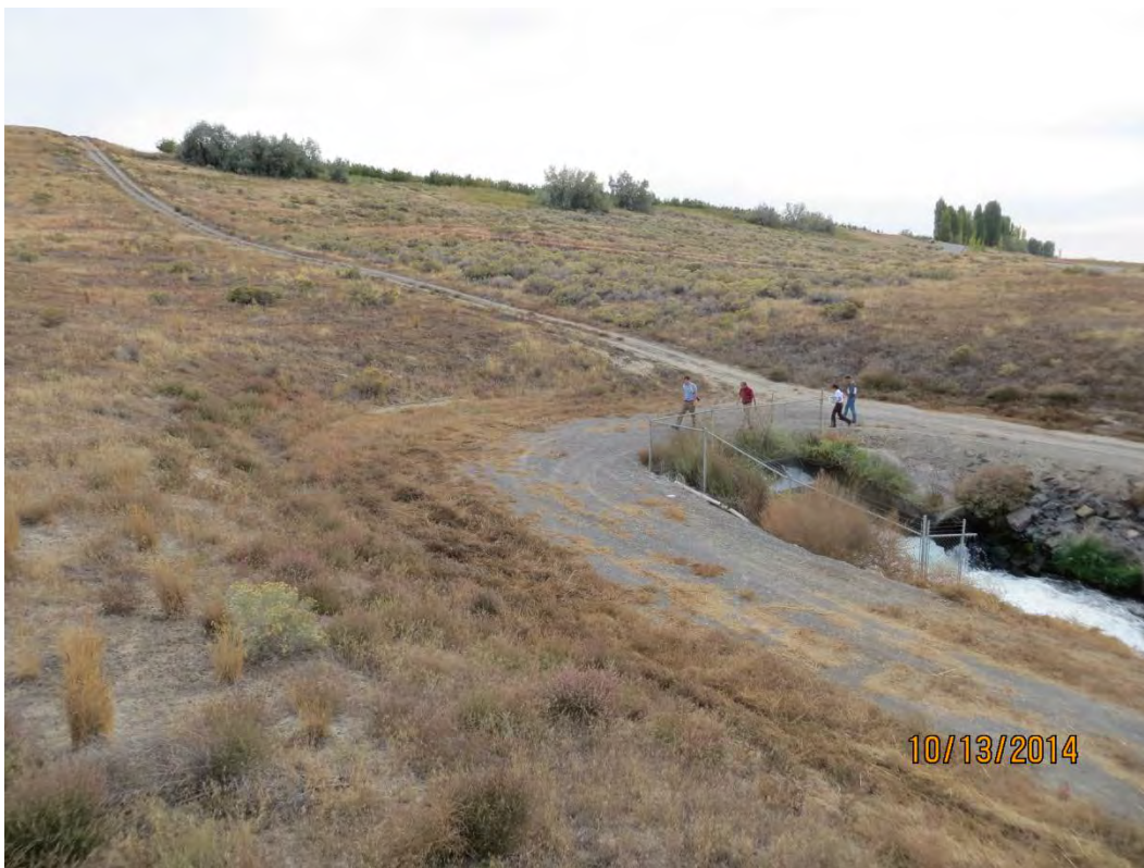
PHOTO 4 BURIED CHUTE AND STILLING POOL LOOKING UPSTREAM
