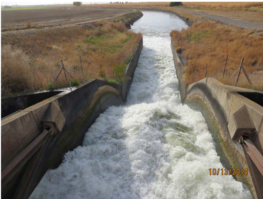
PHOTO 4 CHECK DROP AND STILLING POOL
