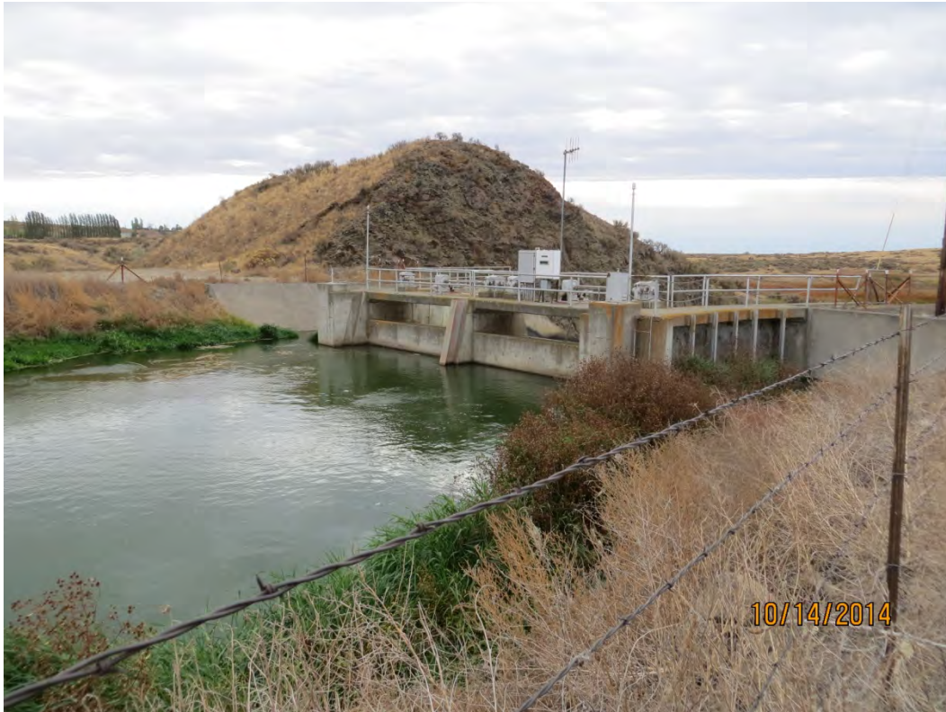
PHOTO 1 INTAKE FOR RADIAL GATE CHECK DROP
