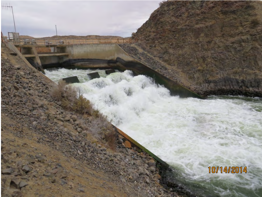
PHOTO 2 DOWNSTREAM END OF CHECK DROP
