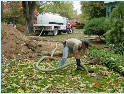
Septic System Pump-out
