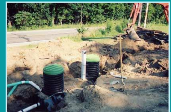
Alternative On-site Sewage Disposal System
