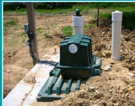
Alternative On-site Sewage Disposal System
