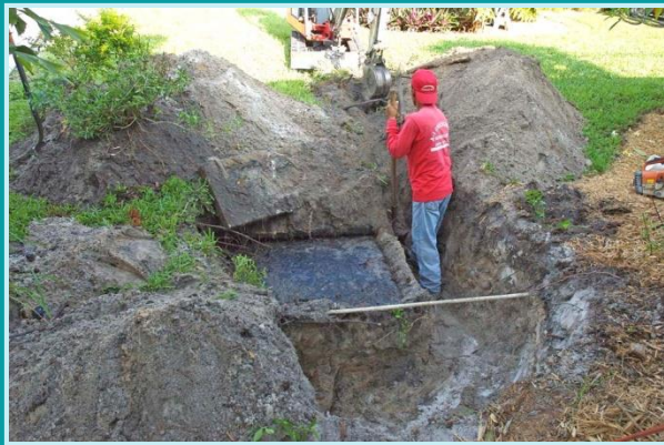
Septic System Repair
