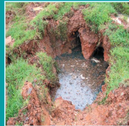
Failed Septic System
