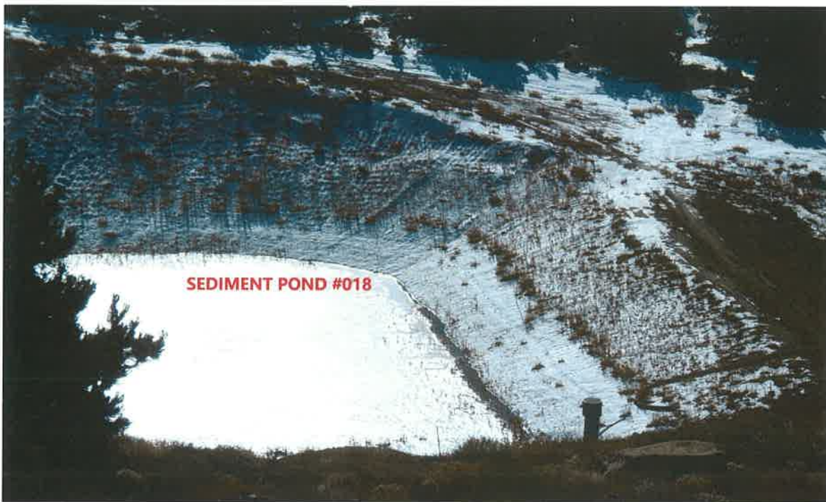
Sediment Pond 018, located west of Sed Trap #1 – photo looking southerly January 12, 2018 No discharge in 2017
