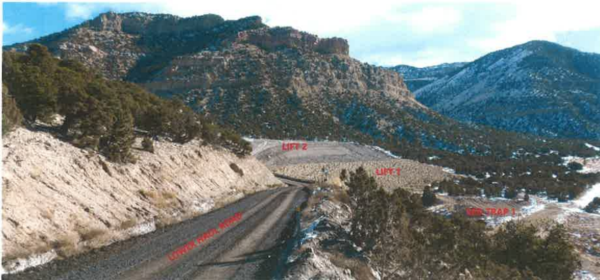
SCA#2 Ash Landfill –looking easterly
