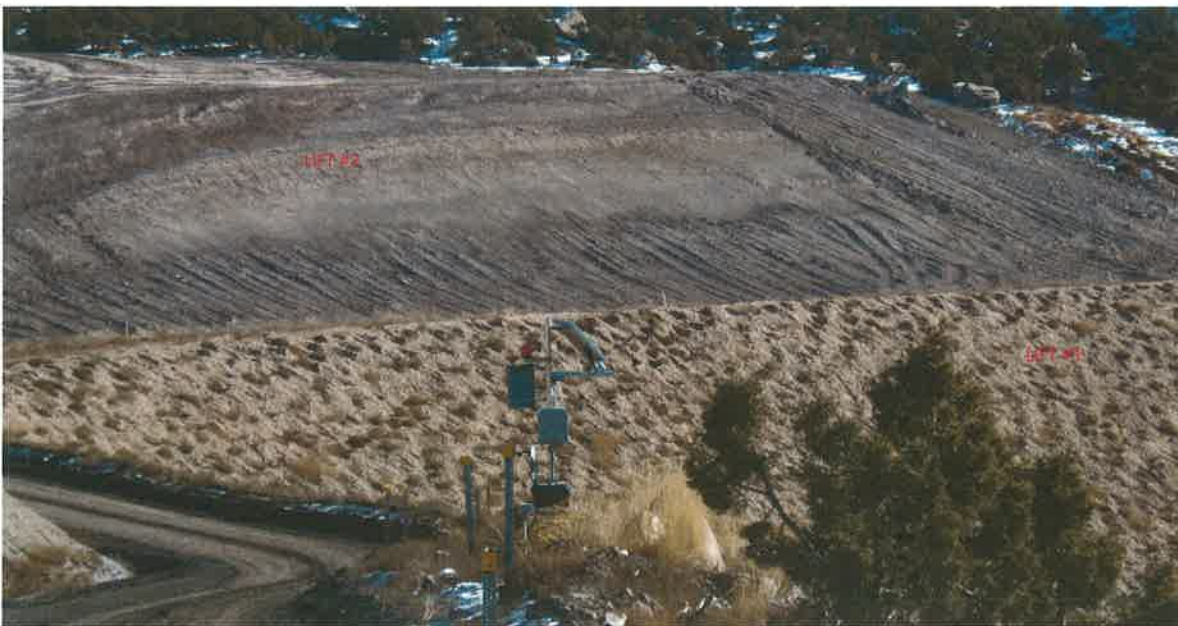
SCA#2 Ash Landfill – lower face looking easterly Lift #1 covered and seeded, vegetation is growing. Lift #2 in process
