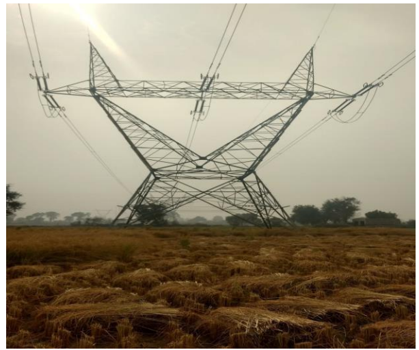
Fig. 8: Site of Broad Base Single Circuit (Multiple Conductors) at Mayer (Hisar)
