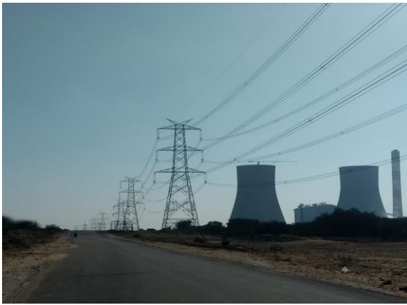
Fig. 14: Site of Broad Base Double Circuit (Multiple Conductors) at Suratgarh Road
