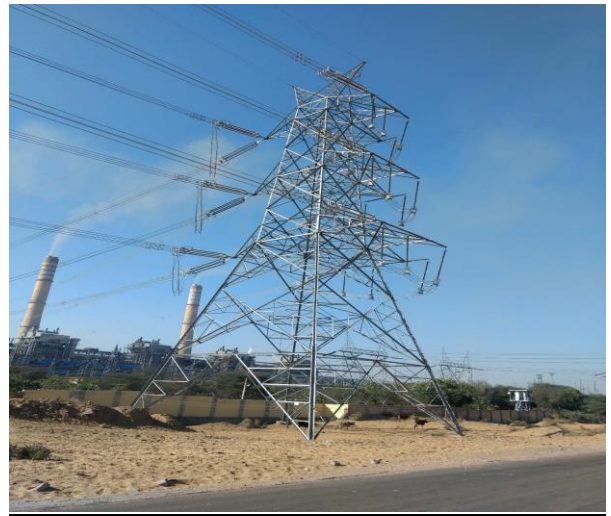
Fig. 12: Site of Broad Base Double Circuit at Suratgarh Road
