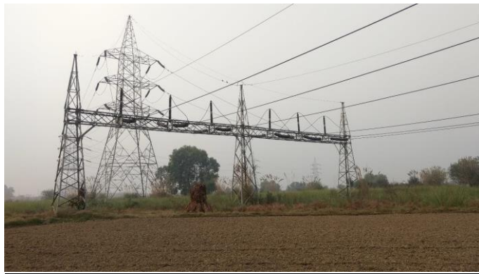
Fig. 9 & 10: Site of Chainnet Structure Double Circuit at Sampla (Rohtak) with vertical and horizontal configurations respectively.
