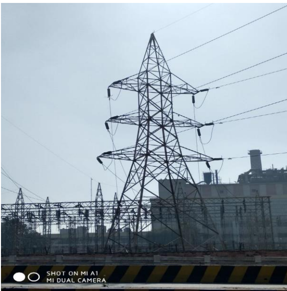
Fig. 3: Site of Single Circuit Broad Base Circuit at Bhatinda- Dabwali Road
