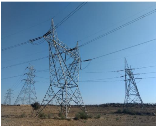
Fig. 11: Site of Broad Base Single Circuit at Suratgarh Road
