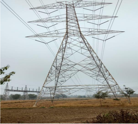
Fig. 5: Site of Broad Base Double Circuit (Multiple Conductors) at Sampla (Rohtak)
