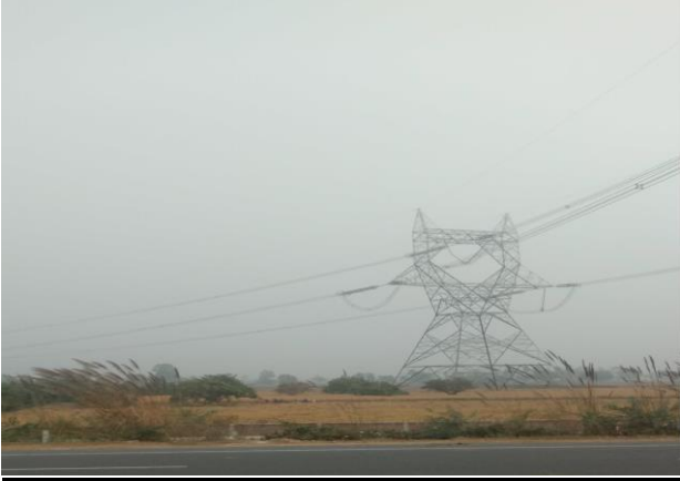
Fig. 13: Site of Broad Base Single Circuit (Multiple Conductors) at Rohtak
