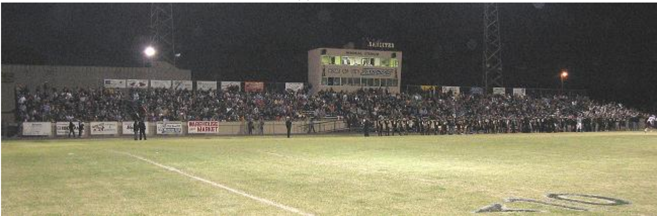
The "Before" picture of Sand Springs Memorial Stadium prior to a well deserved 4 million dollar end of season rebuilding project. Photo/JTBC
