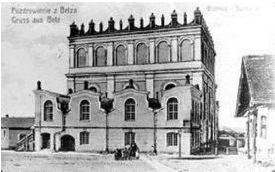
The synagogue in Belz, dedicated in 1843, destroyed by the Nazis during World War II , and demolished in the 1950s.
