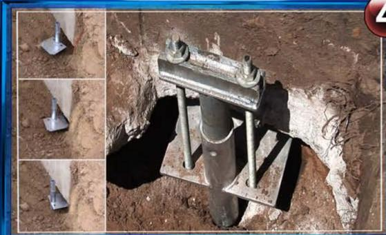
The Tru-Lift® bracket is then installed on each pile and securely attached to the foundation.
