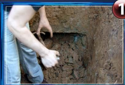
We begin by excavating down to the footing at each pier location.
