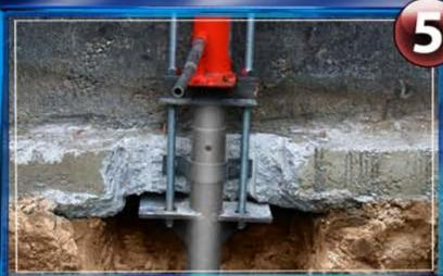
The foundation is raised to the determined elevation and the foundation is permanently stabilized.
