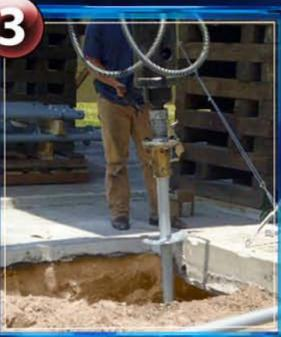
A hydraulic torque drive is used to screw each pier into stable sub soil until design depth is achieved.
