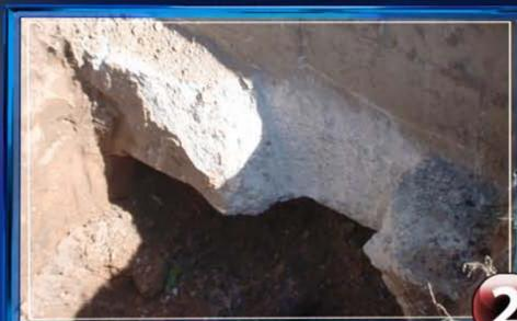
The footing must then be notched to accommodate the Tru-Lift® Bracket
