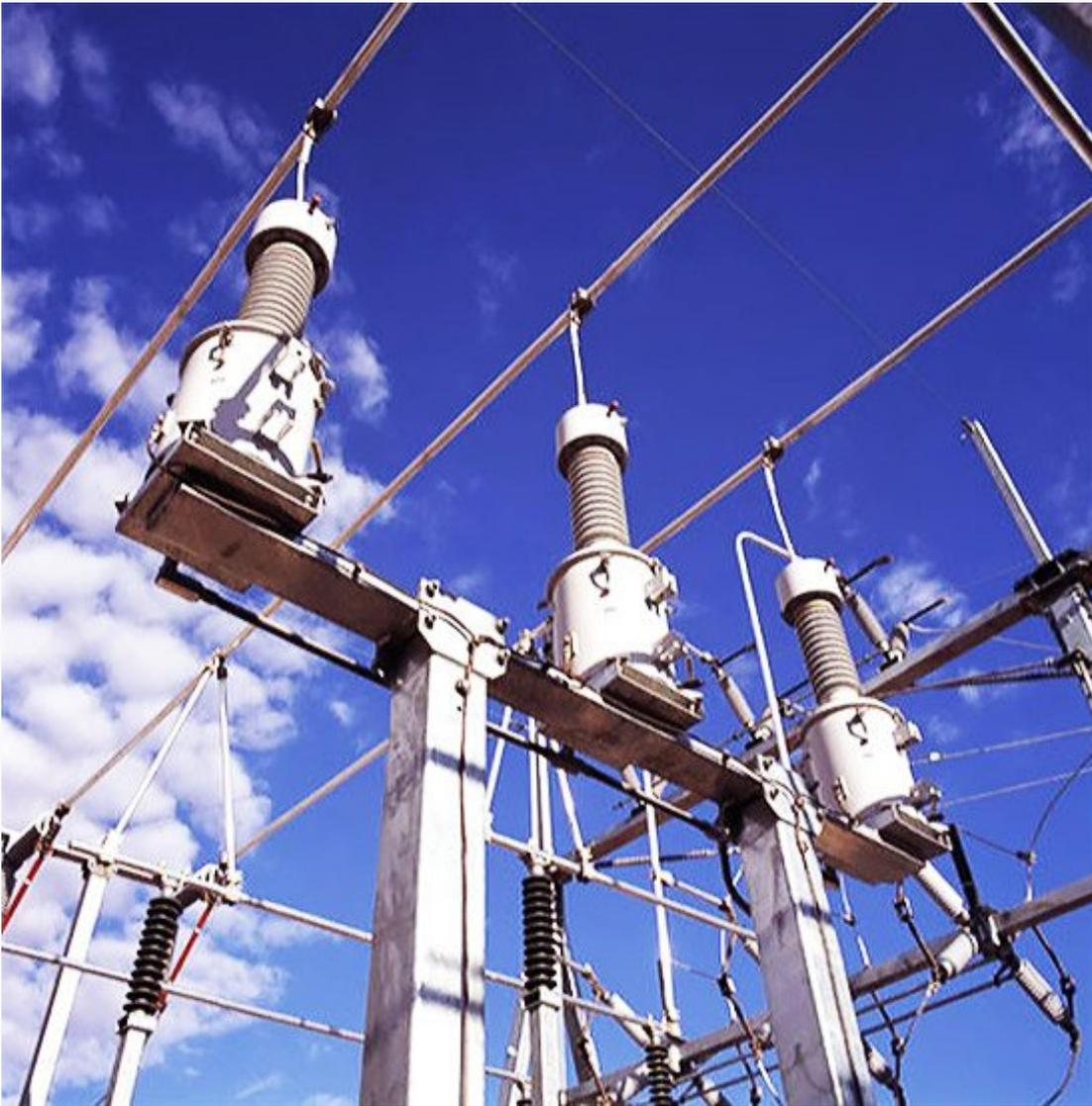
Figure 5 – Outdoor switchgear busbar (upper conductors) with voltage transformers
