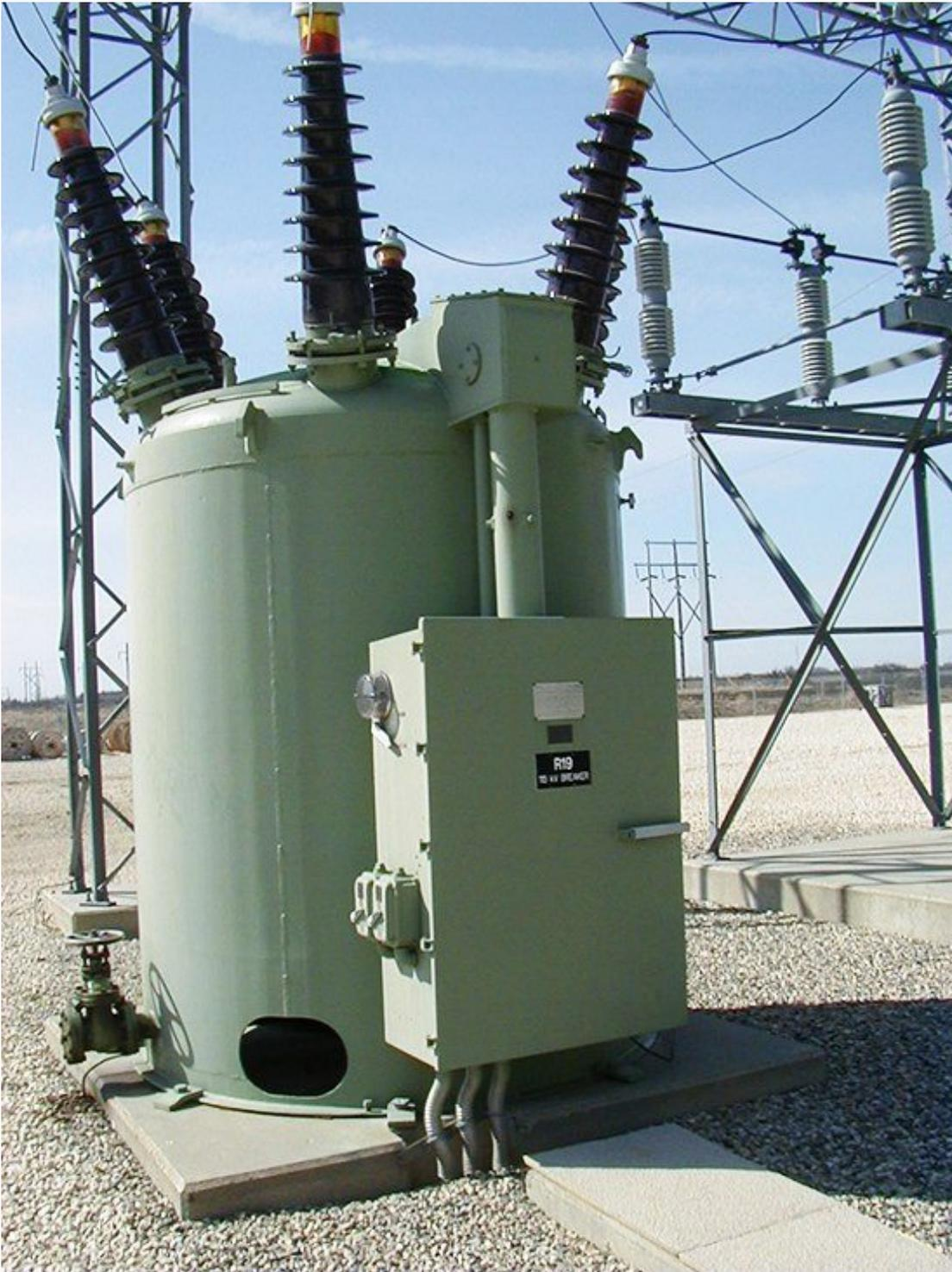
Figure 7 – Outdoor medium voltage oil-immersed circuit breaker
