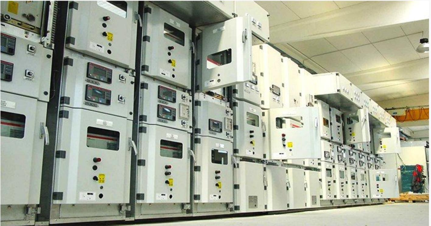
Figure 6 – Air-insulated primary switchgear equipped with Feeder Terminals (type 'UniGear ZS1')
