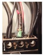
Time marches on and so do its offspring: heat and corrosion. Steve said the owner was lucky that only the wire and not the entire box burned.
