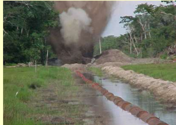
Blasting work on a pipeline in remote Bolivia
