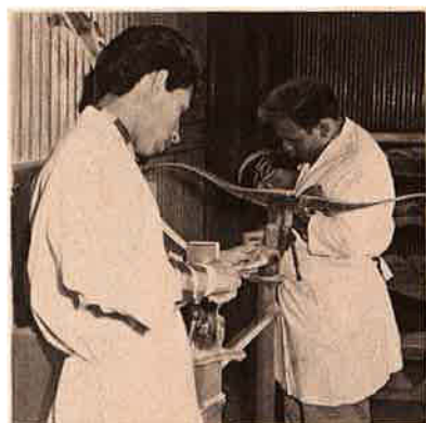
With all the production machines, it is still impossible to achieve Custom quality without the individual touch. Here we see the custom hand shaping of the nocks and overdraw, and the finishing of a PRESENTATION on the contour sander.
