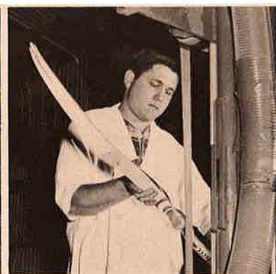
With all the production machines, it is still impossible to achieve Custom quality without the individual touch. Here we see the custom hand shaping of the nocks and overdraw, and the finishing of a PRESENTATION on the contour sander.
