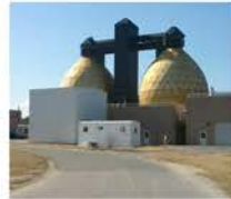
HY-TEK Bio R&D Facility
