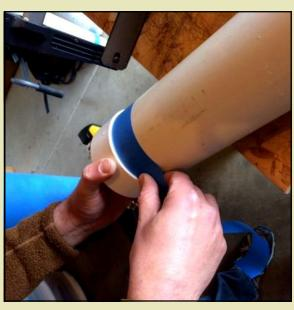
3. Put the cap in place dry and wrap painter's tape around the tube above it, to mark the tube and protect it from the cement. Remove the cap for Step 4.
