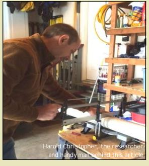
2. Cut the PVC pipe with a fine-toothed saw and sand off the rough edges.
