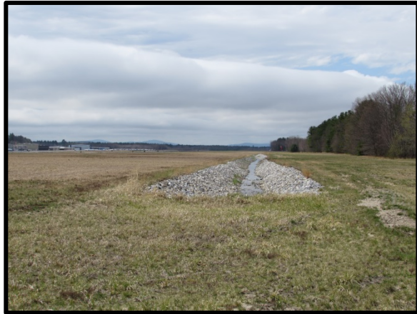
Standing water in drainage swale
