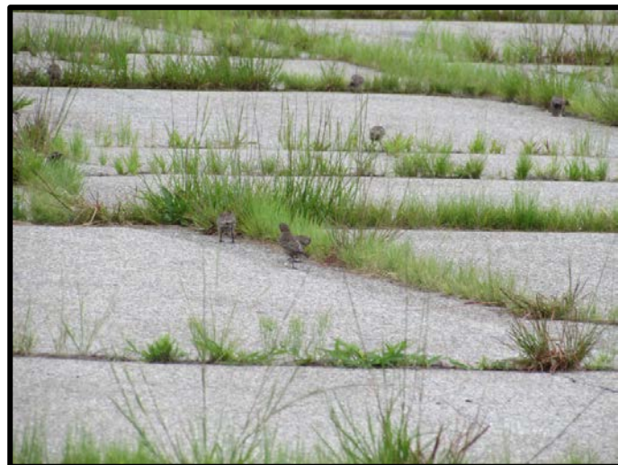
Grass growing through pavement at Boire Field
