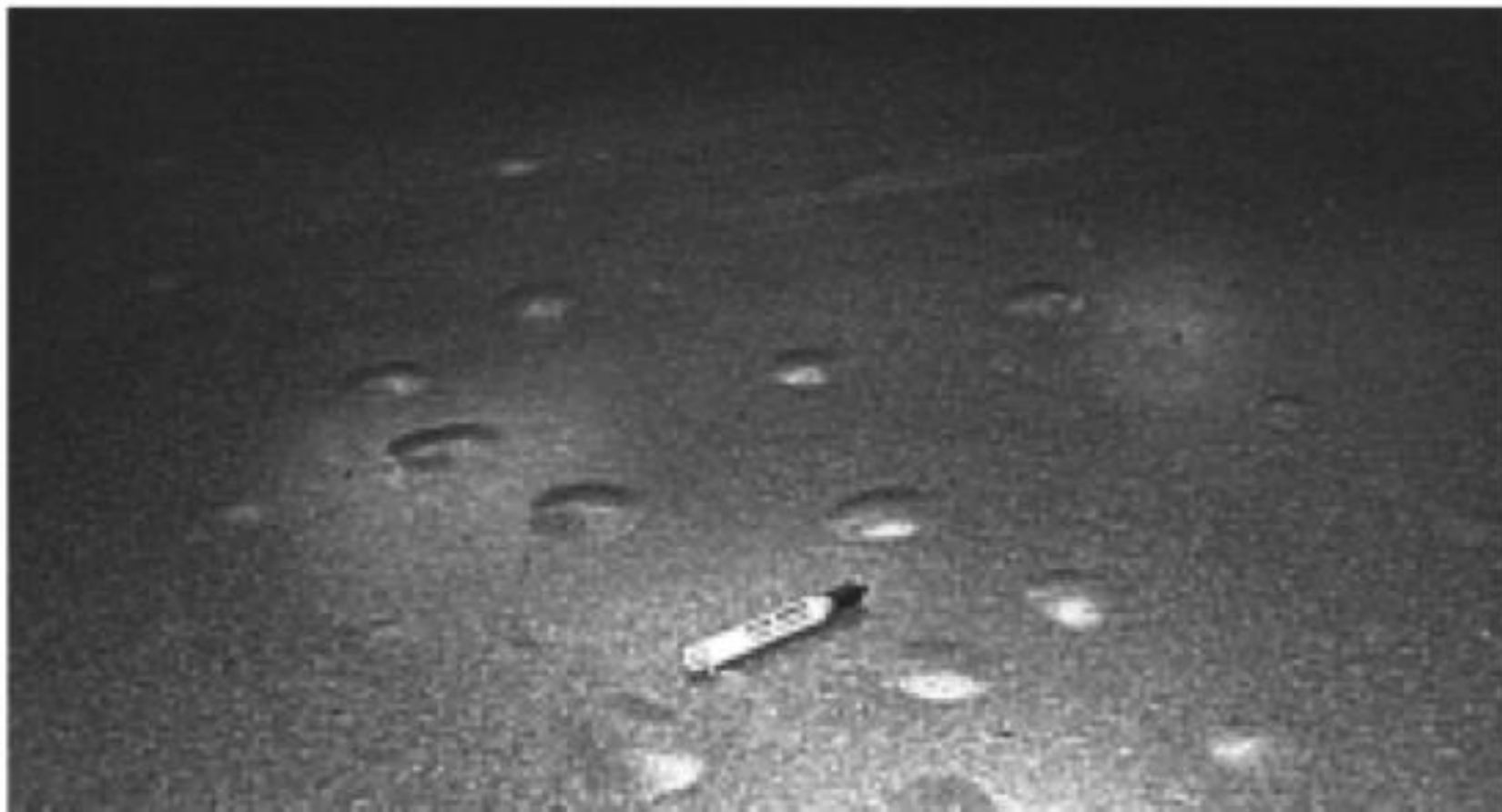
Fig. 1.2—Blisters due to moisture in concrete. (Courtesy of Peter Craig.)
