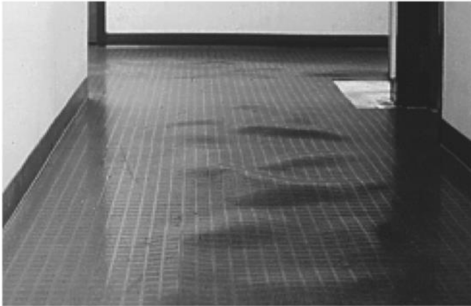
Fig. 1.1—Debonded sheet flooring due to moisture in the concrete slab. (Courtesy of Peter Craig and Herman Protze III.)
