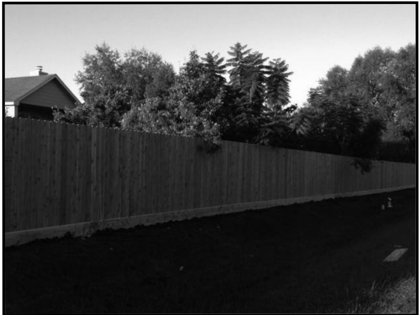
New fence on Florence 8ft.
