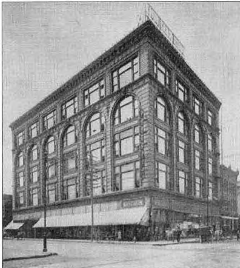
Figure 18, original building, 1904, view northwest from the corner of Walnut and 7 th streets
