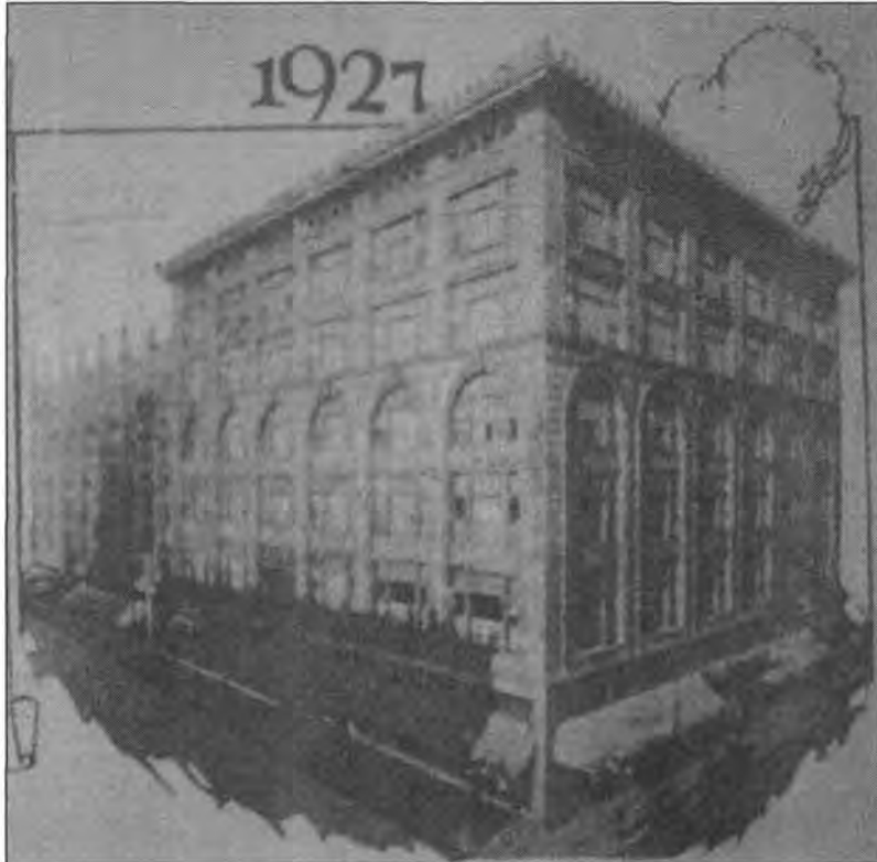
Figure 40; Younkers Building at the time of the 1927 merger, view northwest, note cornice ( Tribune , January 1, 1927, left, February 26, 1927, right)
