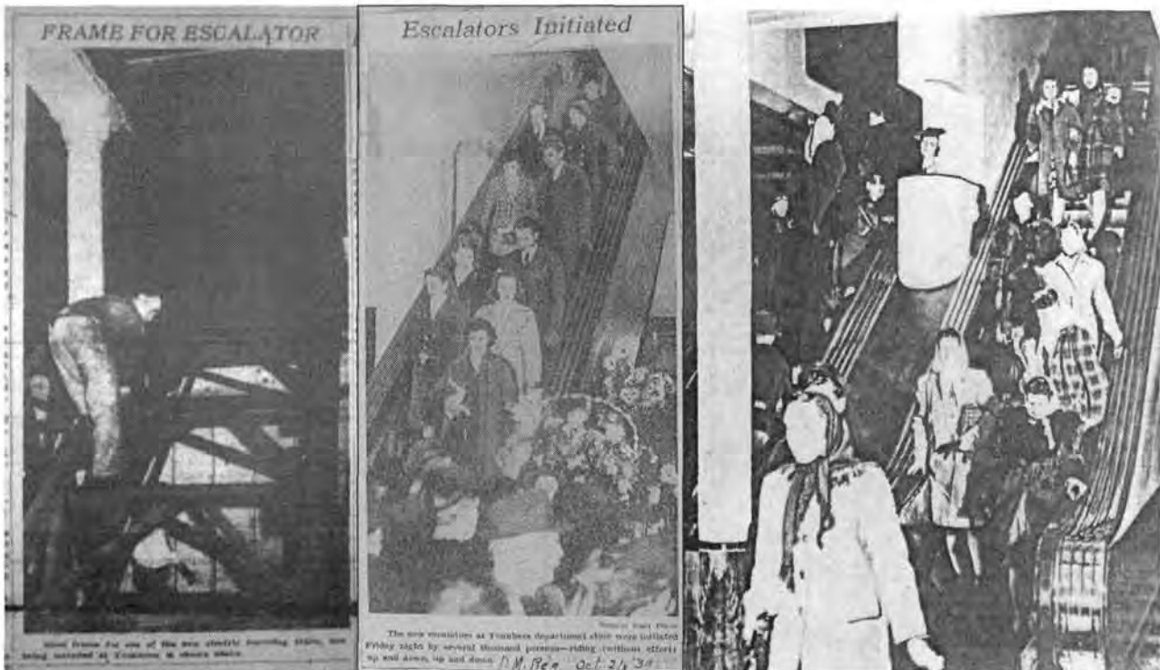
Figure 48: Three escalator images, left to right, installing the frame for the new escalator ( Tribune , June 7, 1939), middle, electric stairway opens, right, in operation 1944 ( Des Moines Register , October 21, 1939; 1944 booklet)
