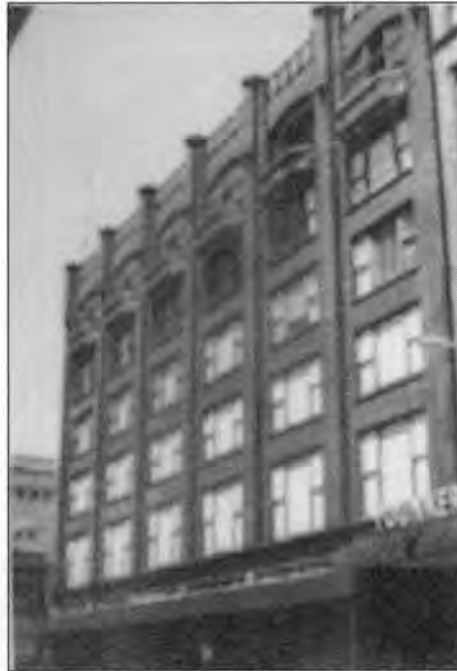
Figure 60: View, Walnut and 8 th streets, looking northwest (SHSI historical inventory photo, either from the Elmet's Windshield Survey, 1974)
