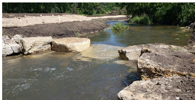
Streambank stabilization
