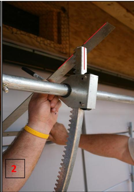
With all Shutter Units hanging freely and in the exact same near closed position, firmly tighten down both set screws with a 4mm Allen wrench while the Pinion is positioned on the marks. Continue this procedure for each Pinion.
