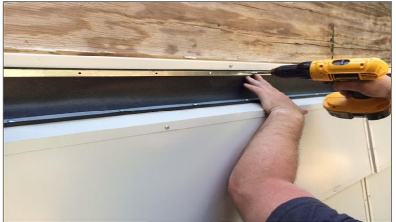
Next, fasten a screw through both overlapping seals to secure them to the Vertical Rails and also at each end rail. Update: Use Large Washer under screw head. Washer provided with hardware. **Do Not over tighten causing damage to the seal.**
