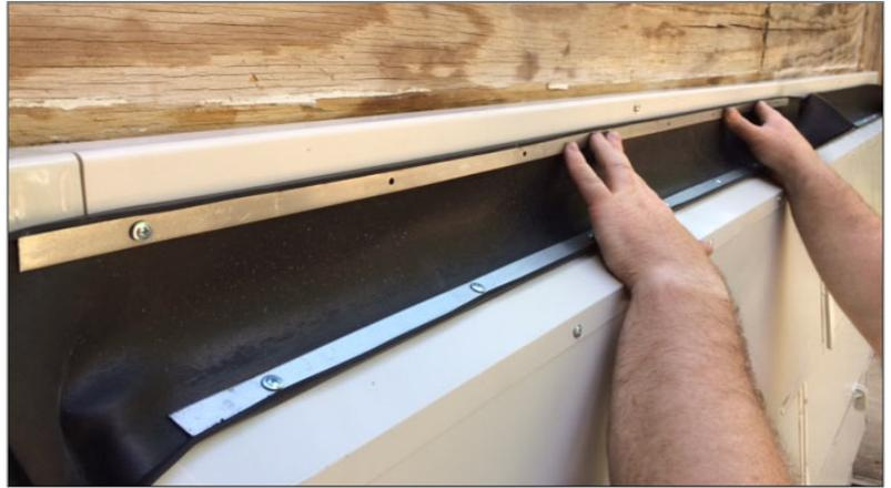
Fasten the Retainer Strip with screws to the flat face of the Top Rail just below its center screw. The ends of the Retainer should be placed at the middle of each Top Coupler.
