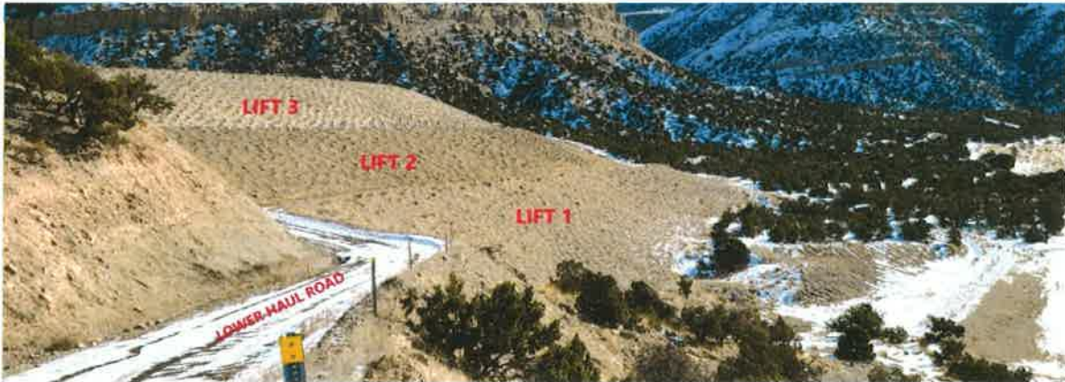
SCA#2 Ash Landfill –looking southeasterly
