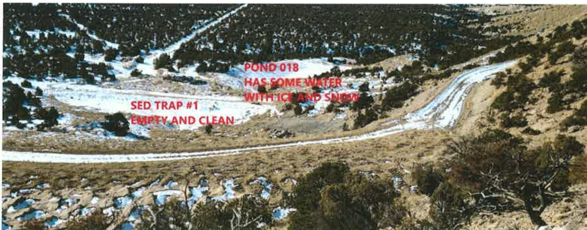
Sediment Pond 018, located west of Sed Trap #1 – photo looking westerly
