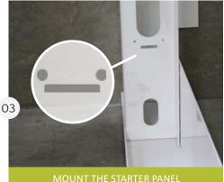
Insert the STARTER (L) PANEL (fluorescent green label) into the BOTTOM RAIL in the correct position. The rectangular slots located on the sides of the panels should sit below the two screw holes, as shown above.
