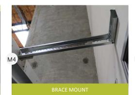
BRACE MOUNTS (pastel blue label) are fastened to TOP RAILS and mounted to an existing wall structure. Use as frequently as possible.
