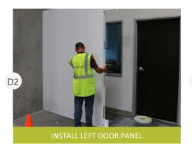
Insert the LEFT DOOR PANEL (fluorescent orange/yellow) into the BOTTOM RAIL. Slide flush against the PANEL and fasten.
