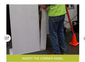
Insert the CORNER PANEL (fluorescent red label) into the CORNER BOTTOM RAIL (if applicable) and fasten. Continue adding PANELS as shown in step 6.
