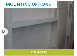
STIFFENERS (pastel yellow label) provide track for wires. Install between PANEL cutouts and secure; flanges must point upward. \**Not all walls require these.*
