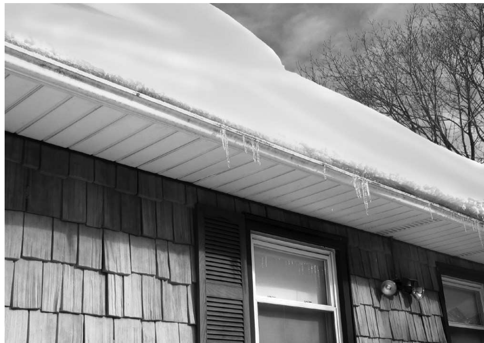
Heavy snow loads and movement when snow melts can cause problems on your roof. Call in a professional when whether permits and get damaged shingles repaired or replaced.
