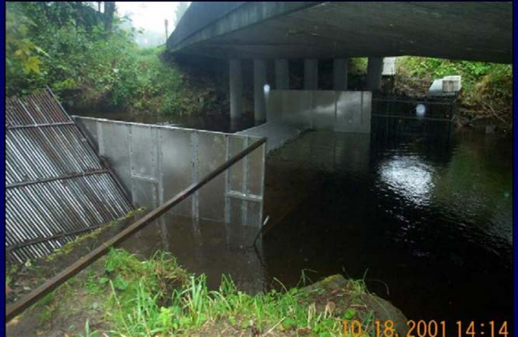
Umbrella Creek Resistance Board Weir and Adult Sockeye Trap
