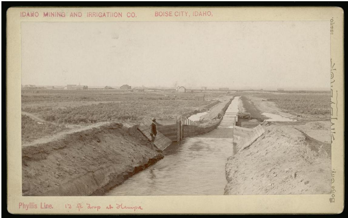
**Figure 2 Phyllis Line, 13-foot Drop at Nampa, c. 1890**
