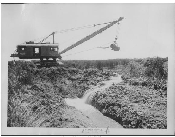
Figure 22 June 22, 1914 Electric Dredge excavating, Purdam Slough Drain on Lemp's Ranch." <sup>108</sup>
