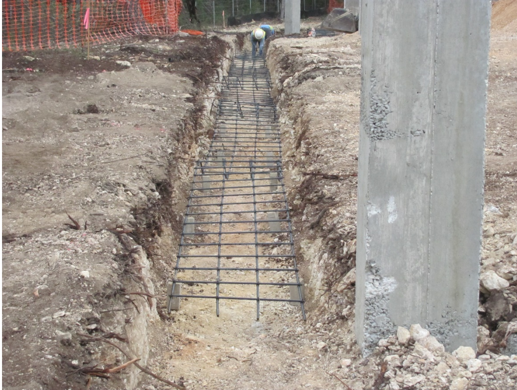
EXHIBIT 5 – RETAINING WALL REBAR 11.10.20
