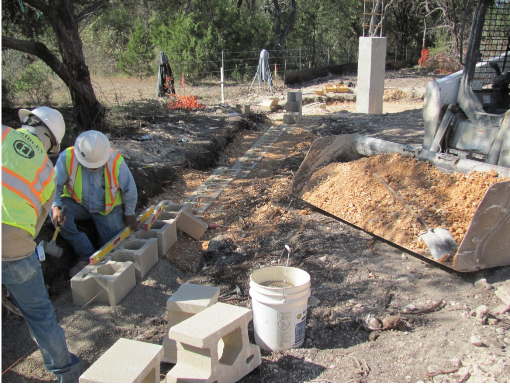
EXHIBIT 9 – RETAINING WALL CONSTRUCTION 11.18.20
