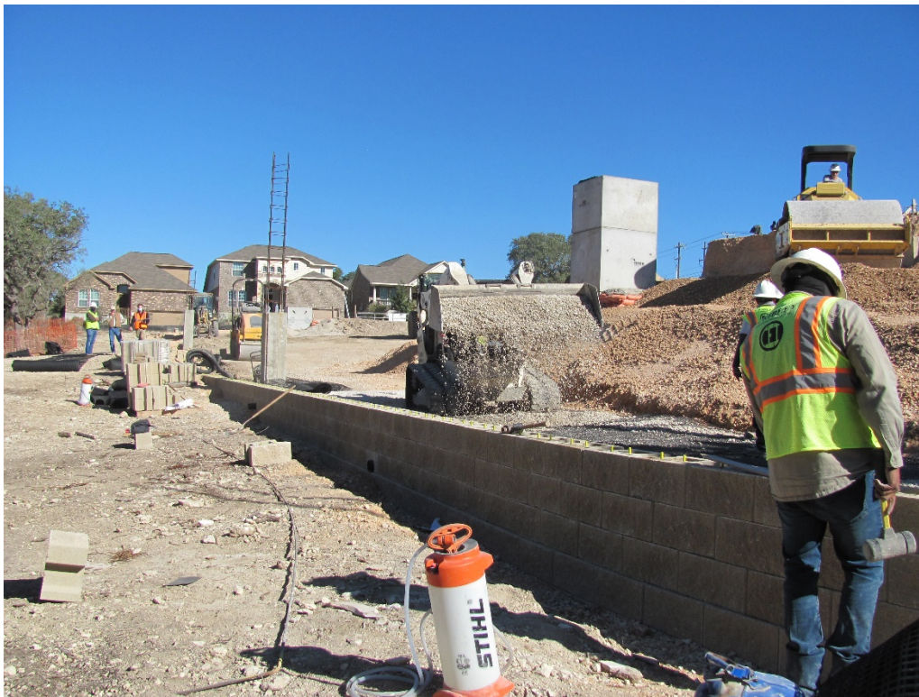
EXHIBIT 14 – RETAINING WALL CONSTRUCTION 12.07.20
