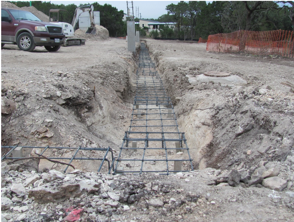
EXHIBIT 6 – RETAINING WALL REBAR 11.12.20
