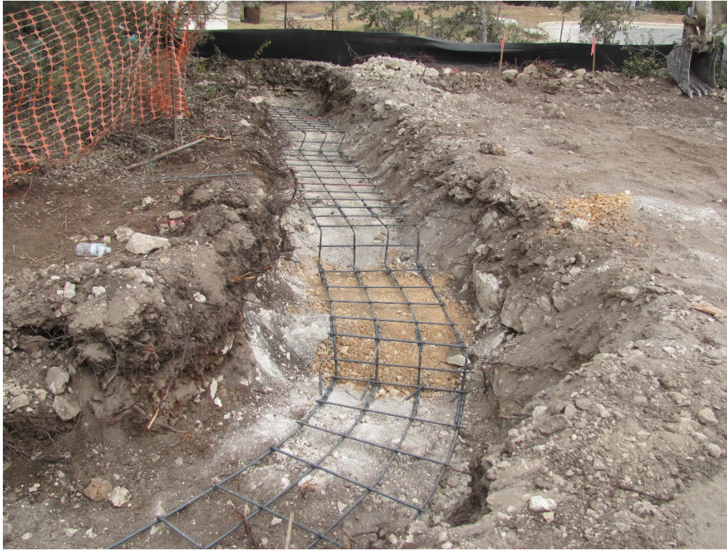
EXHIBIT 7 – RETAINING WALL REBAR 11.13.20
