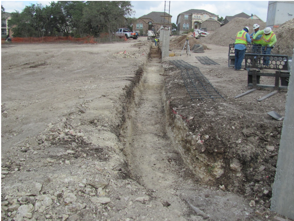
EXHIBIT 4 – RETAINING WALL EXCAVATION 11.09.20
