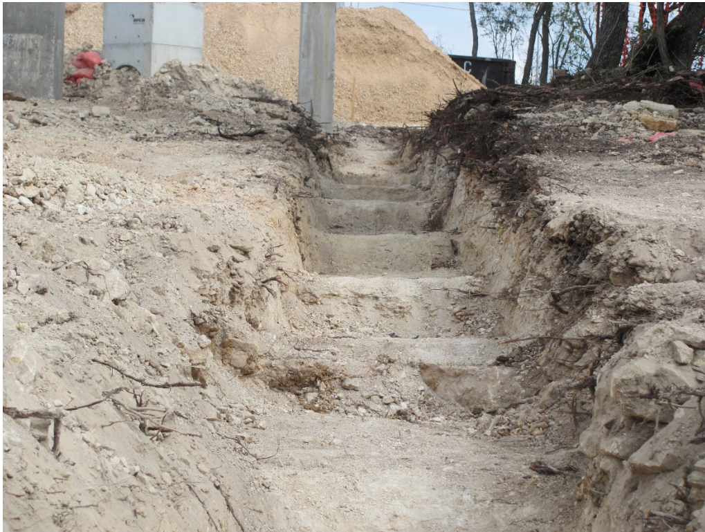
EXHIBIT 2 – RETAINING WALL EXCAVATION 11.06.20
