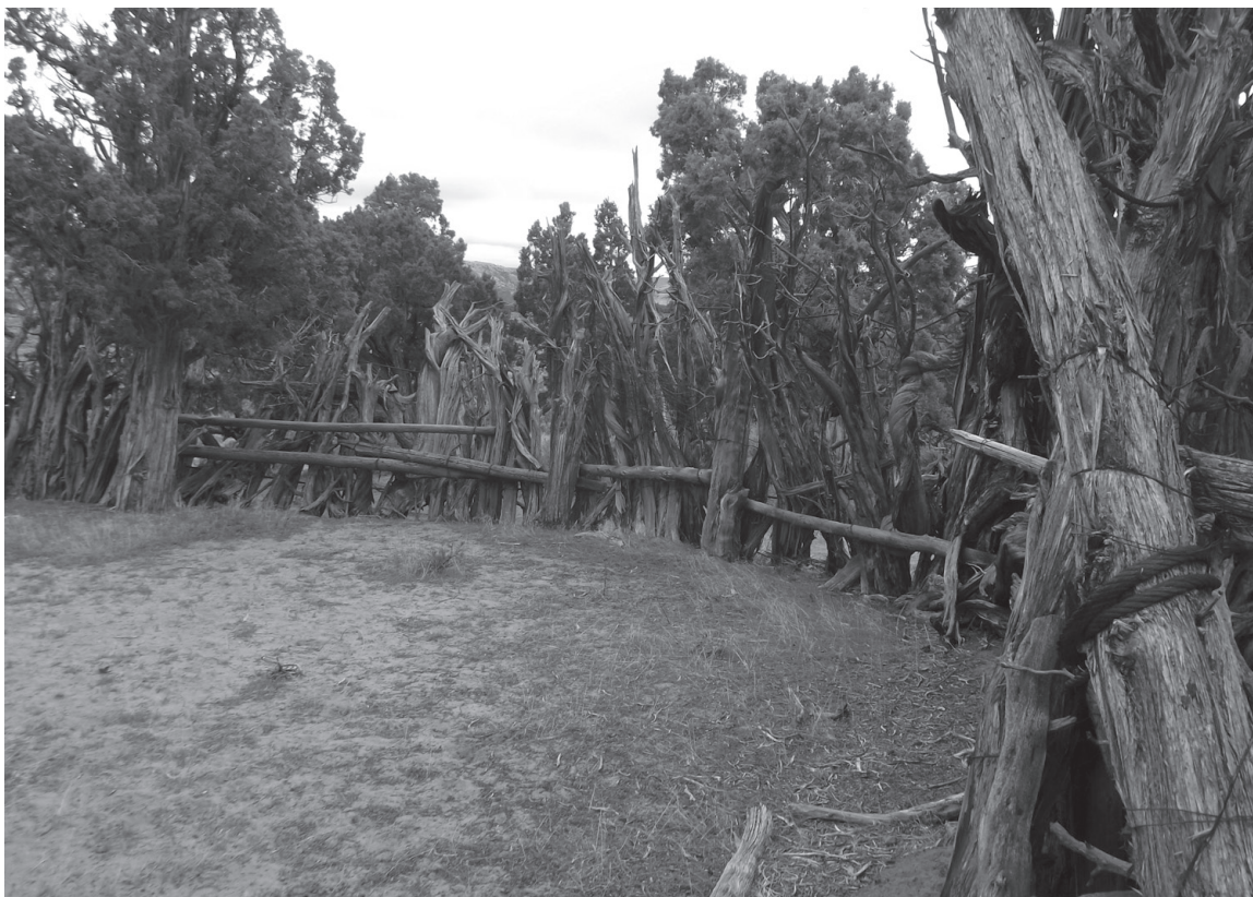
Figure 7: Photograph of inner round corral at Fire Hole Horse Trap showing stockade construction.
