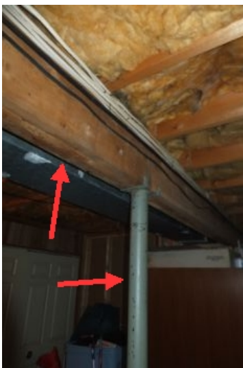
Wood Beam and Steel columns
