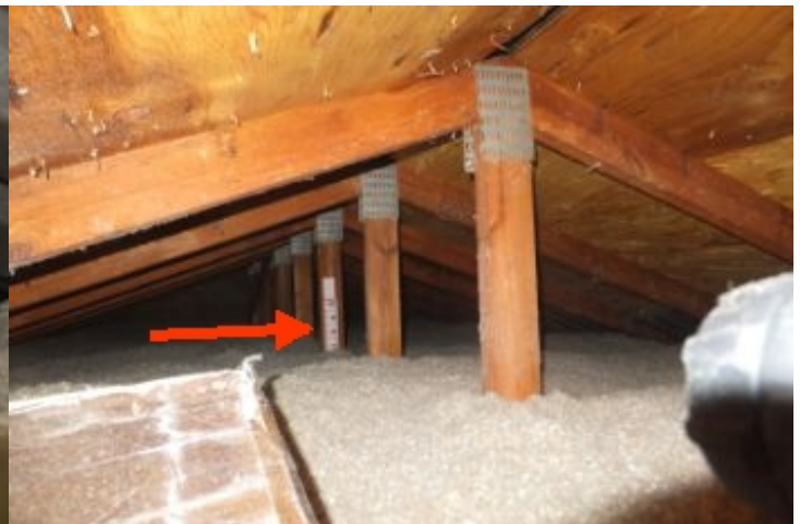
Insulation in 13.5" thick (ruler on truss)
