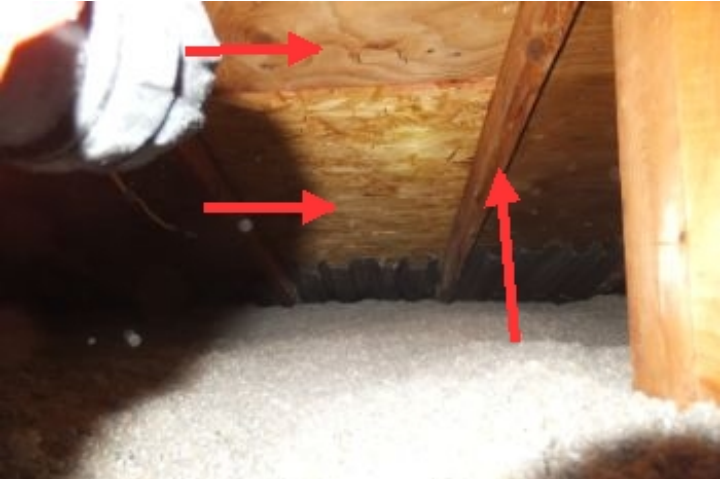
Different Sheathing Types & 2"x4" Trusses
