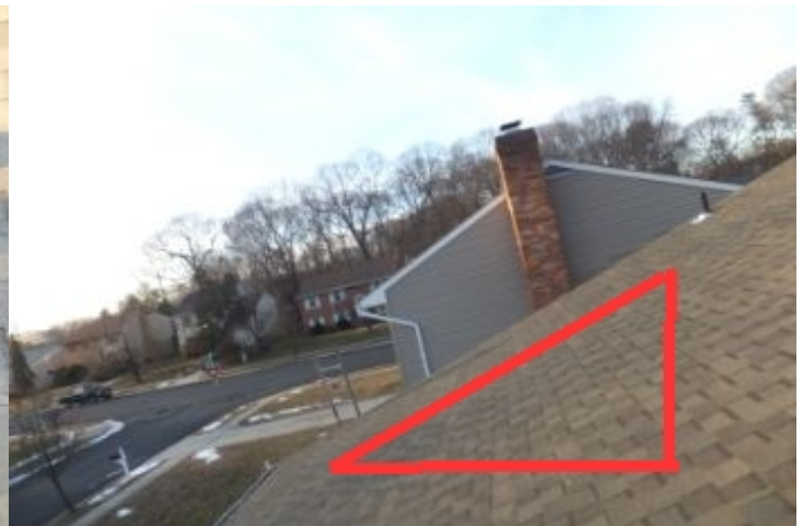
Roof has a 3:12 pitch
