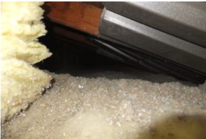
Corrugated sheet system ensuring ventilation
