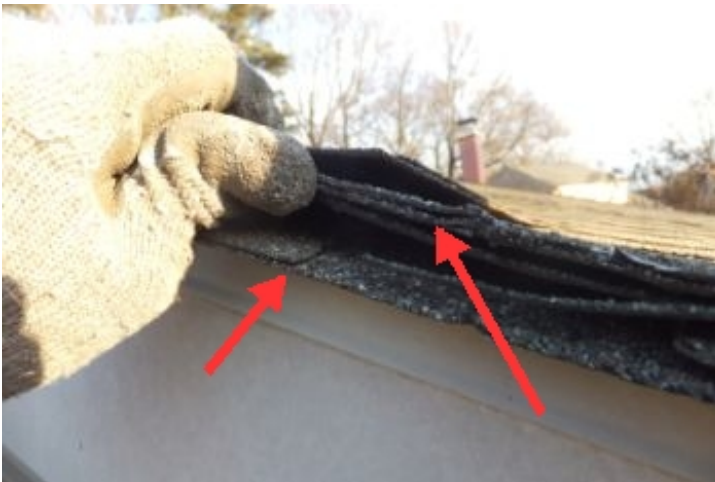
Second layer of shingles
