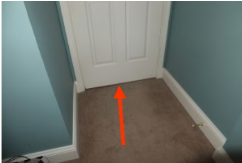
Bedroom doors too tight to floor. Does not allow return air to flow.
