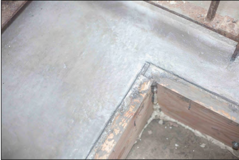
Figure 41: Repaired concrete at landing.
