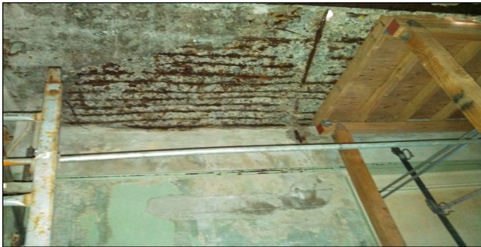
Figure 5: Severe delamination and spalling at the underside of stair landing with approximately 50-60% loss of reinforcement.
