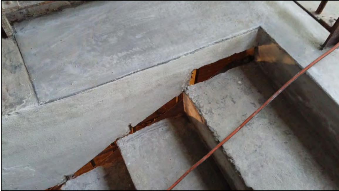
Figure 44: Completed landing/stair connection.
