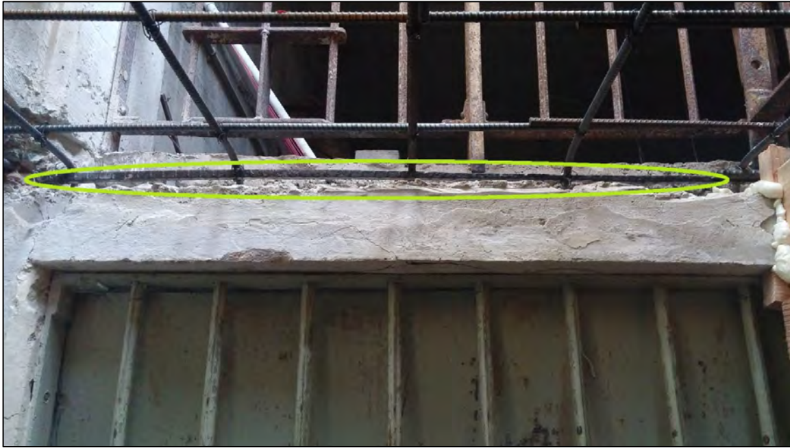
Figure 25: Preserved in situ 5'9" section of steel reinforcing from original construction (circled in yellow).
