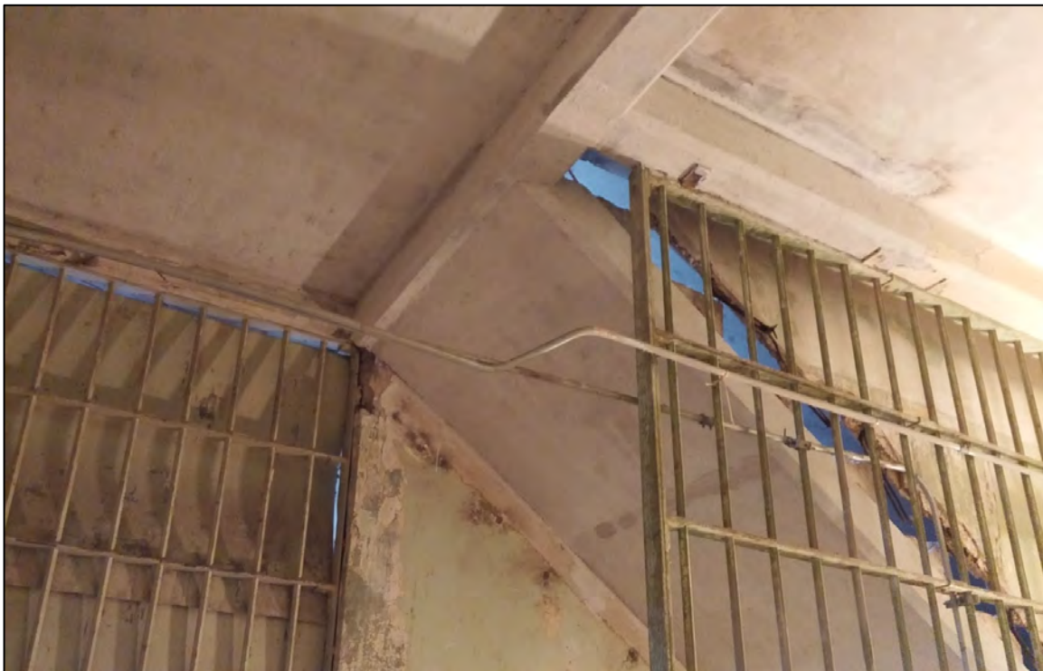
Figure 47: Completed beams, landing, and stair, view from beneath.
