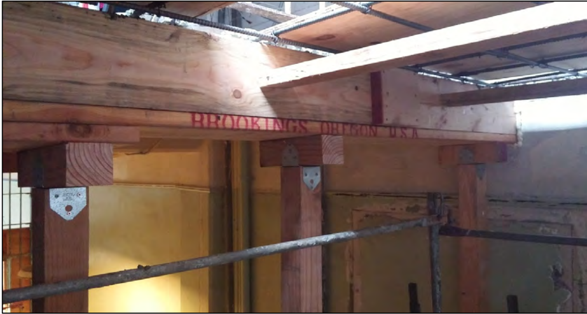
Figure 29: Beam formwork and shoring.
