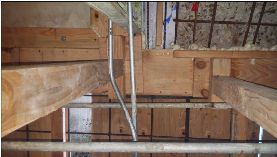
Figure 30: Beam formwork and shoring.
