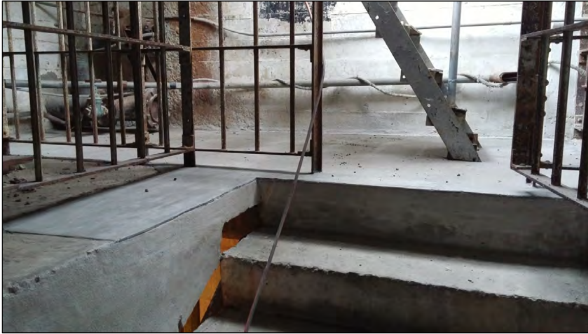
Figure 43: Completed landing.
