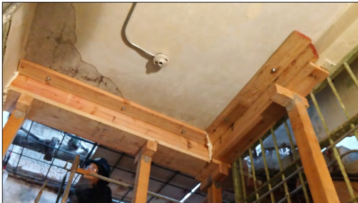
Figure 28: Beam formwork and shoring.
