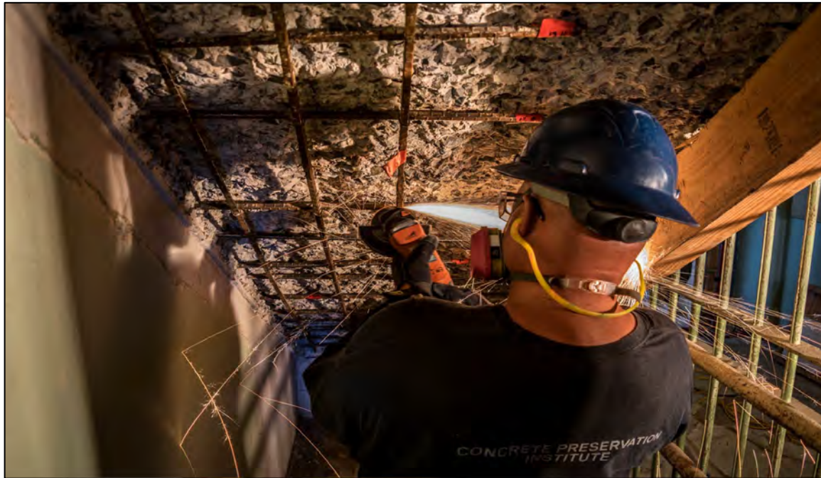
Figure 16: Removal of deteriorated steel reinforcing.
