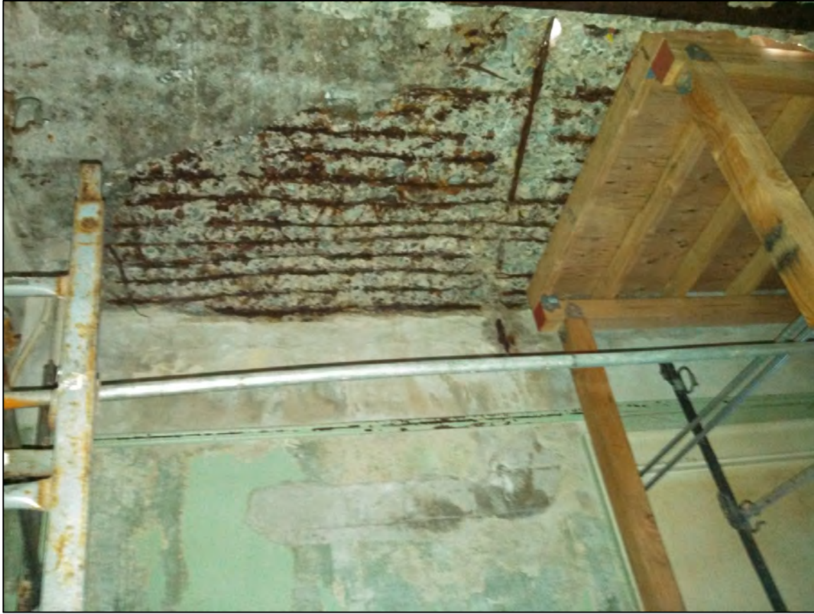
Figure 18: Existing 4" on center, parallel, badly damaged reinforcing steel at landing.
