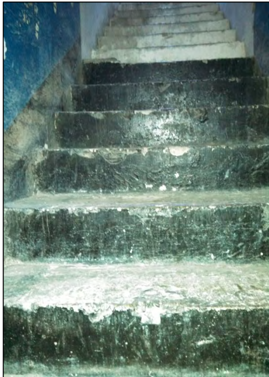
Figure 4: Existing condition of the stairs. The preservation approach was to preserve the treads since they show so much history with their worn appearance. Repairs were done from below. These stairs share the wall with the historically significant graffiti.
