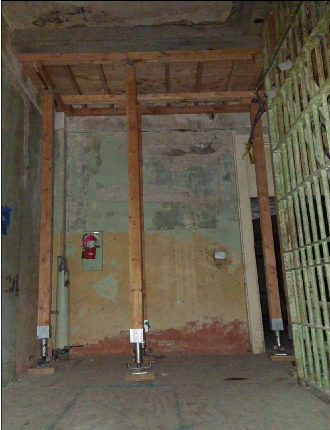
Figure 32: Landing slab shoring and formwork.
