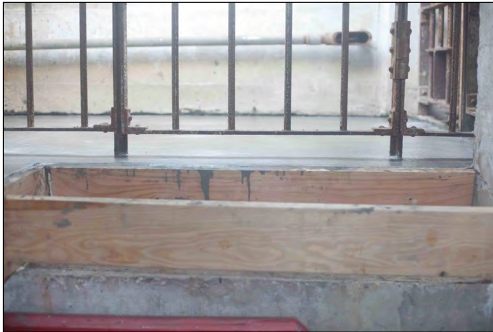
Figure 38: Formwork at landing.
