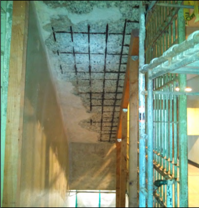
Figure 6: Existing conditions of underside of stairs; extensive delamination due to corrosion of the reinforcing mat.
