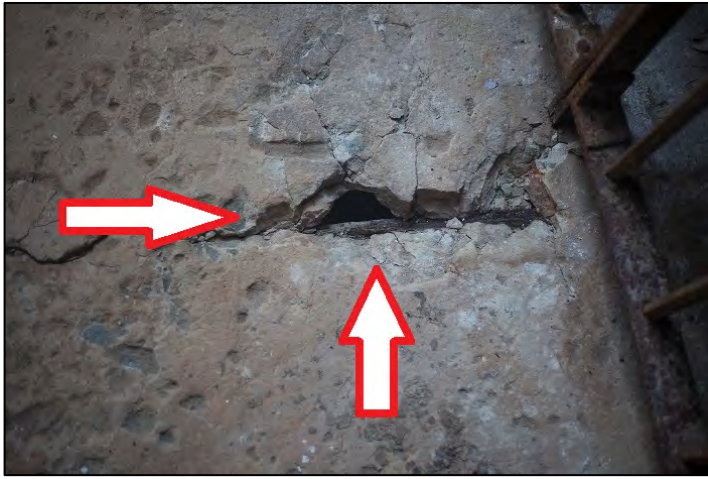
Figure 7: Top surface of the landing showing a void approximately 4" x 3"
