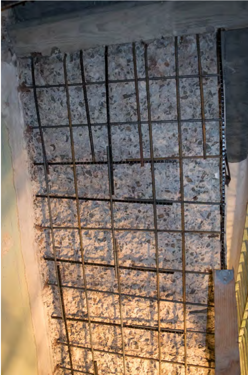
Figure 17: New steel reinforcing spliced onto existing historical reinforcing that was in an adequate condition to be left in place.
