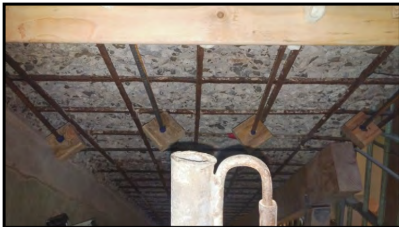
Figure 24: Lower side s-bend lap reinforcing steel at landing connection to stairs.
