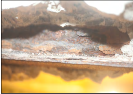
Figure 9: Severe corrosion on the I-beam parallel to the landing.
