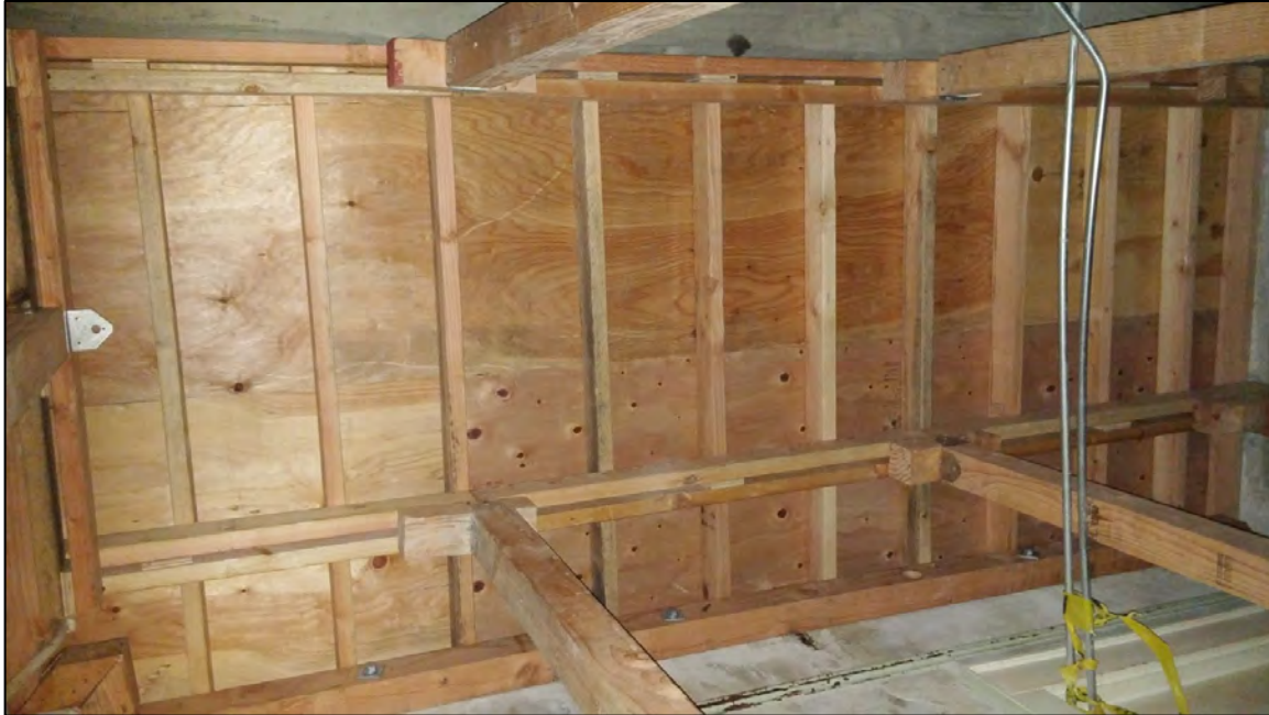
Figure 31: Landing slab formwork, shoring, stiff back, and whalers.
