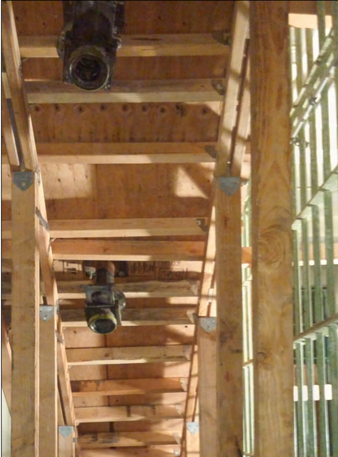
Figure 36: Stair soffit formwork and pump valve positioning.
