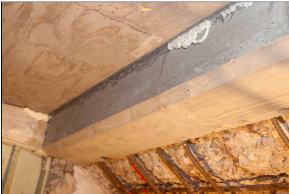
Figure 40: Repaired concrete at landing beam and slab after removal of forms (notice bottom side stairs at below/right/ demolition complete, awaiting formwork and repair).
