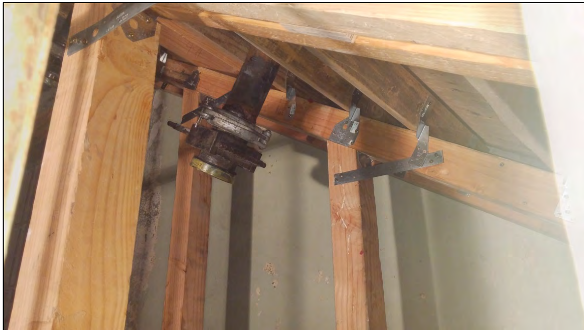
Figure 35: Stair soffit formwork and pump valve positioning.
