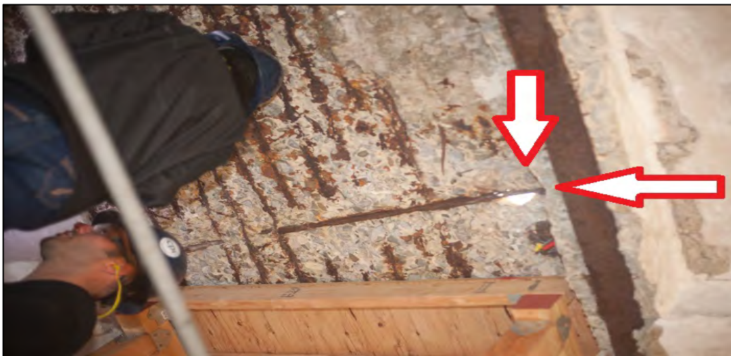
Figure 8: Underside of the landing showing void appearing in Figure 6 as well as general concrete deterioration.
