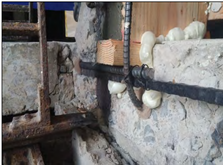
Figure 23: Upper side of s-bend lap reinforcing steel at landing connection to stairs
