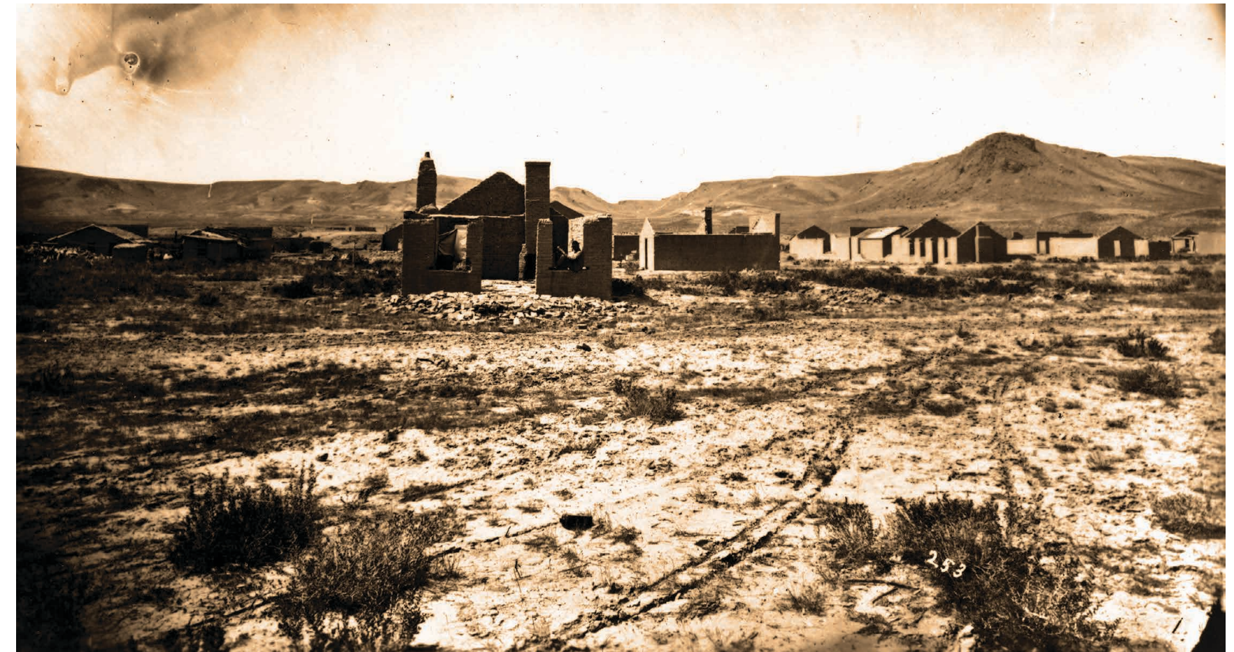
Green River Station, Wyoming. Ruins of adobe houses which were abandoned when construction work on the Union Pacific railroad was moved to another location. 1871 photo by E. O. Beaman on the second Powell expedition.
