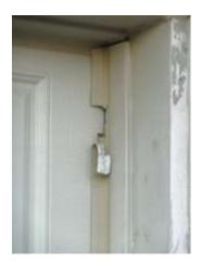
Additional Notes: Torn on right hand side of the garage door, needs be replaced. H. Windows
